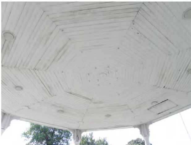
View of Ceiling Looking Southwest
