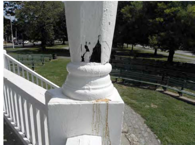
Column #2: Serious Rot on Both Sides of Column; Also Missing Brackets
