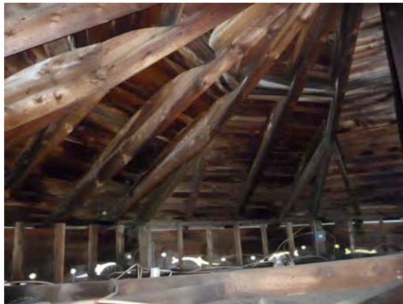
From the Ceiling Hatch Looking at the Northern Roof and Fascia
