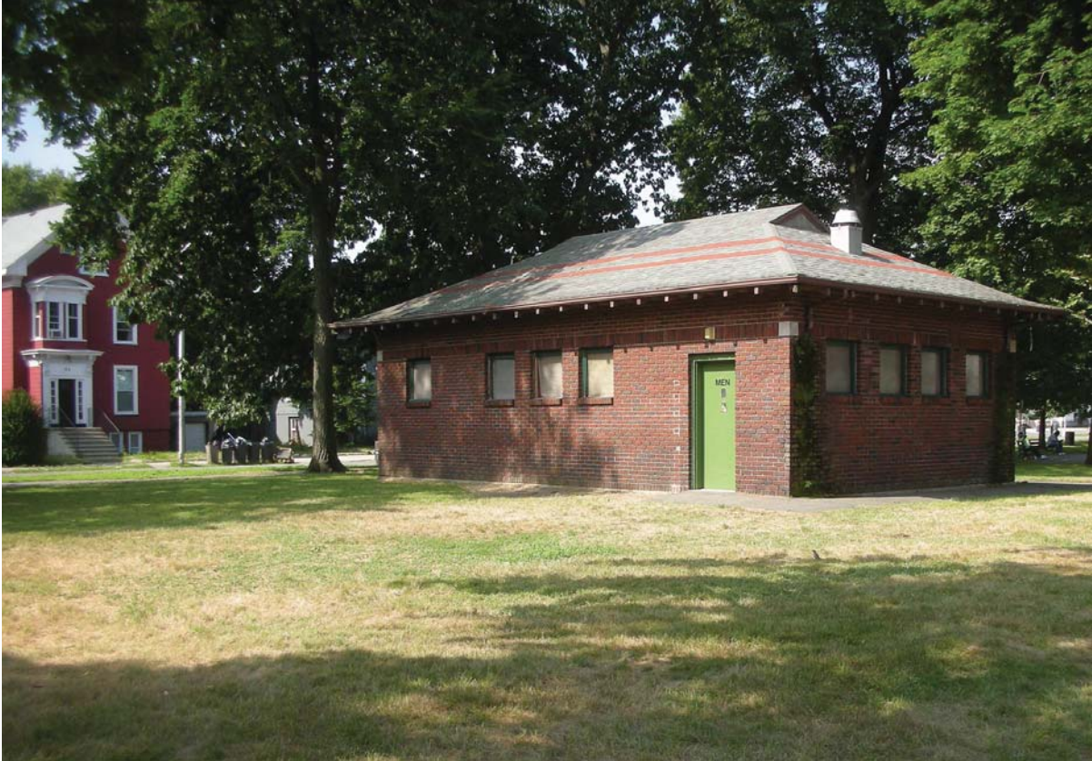
Comfort Station - July 2010
