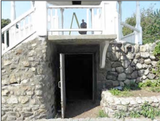
View of Floor Slab Over Basement Doorway
