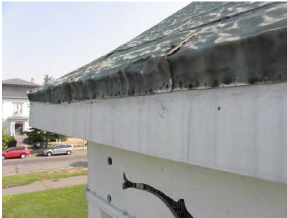
Existing View of Roof Edge without Drip Edge Moldings and Profile
