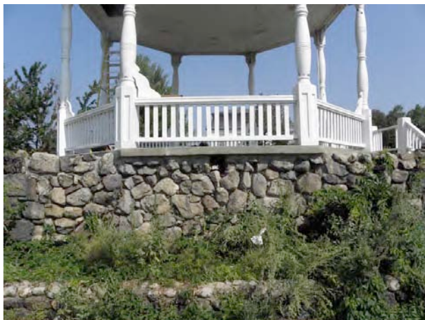
Concrete Pedestals for Wooden Columns on South Side of Bandstand
