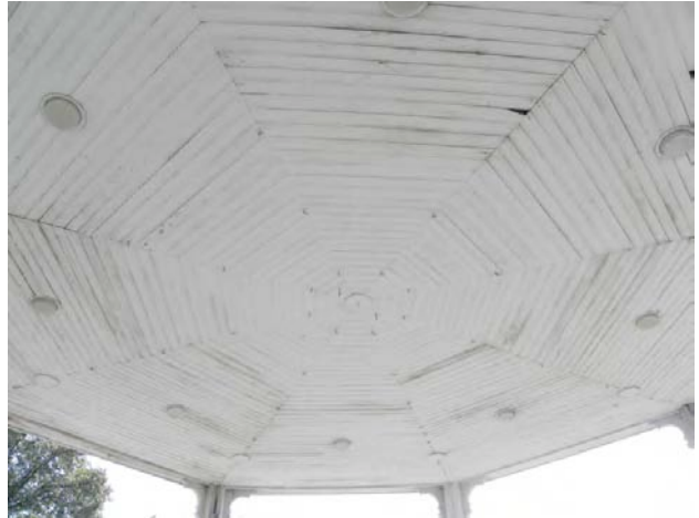
View of Ceiling Looking Southeast
