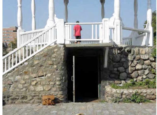
View of Existing Balustrade with Square Balusters, Missing Balusters & Brackets
