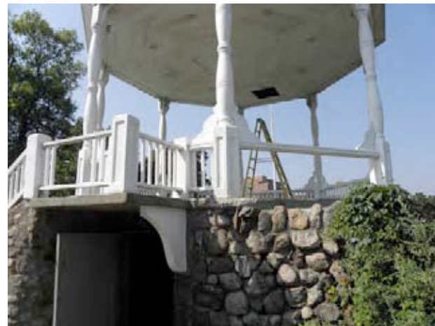
Concrete Pedestals for Stairway Balustrade
