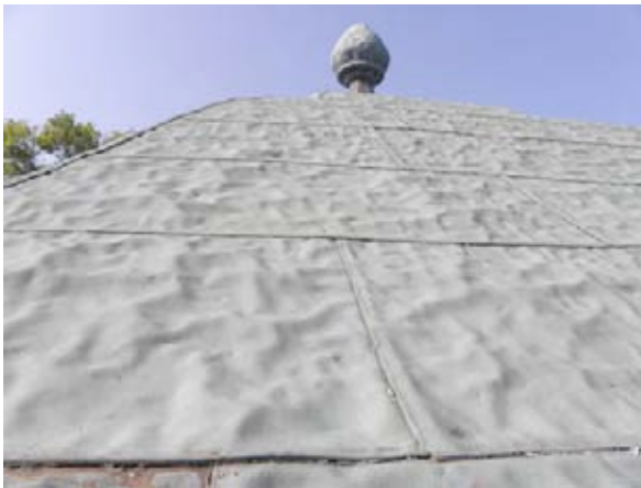
Textured Appearance of Copper Alloy Sheets Joined with Seams
