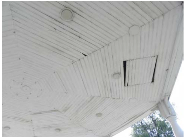
View of Ceiling Hatch Looking South
