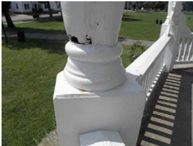
Column #2: Serious Rot on Both Sides of Column; Also Missing Brackets
