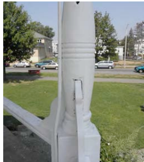
Column #8 Showing Shadow of Larger Original Bracket
