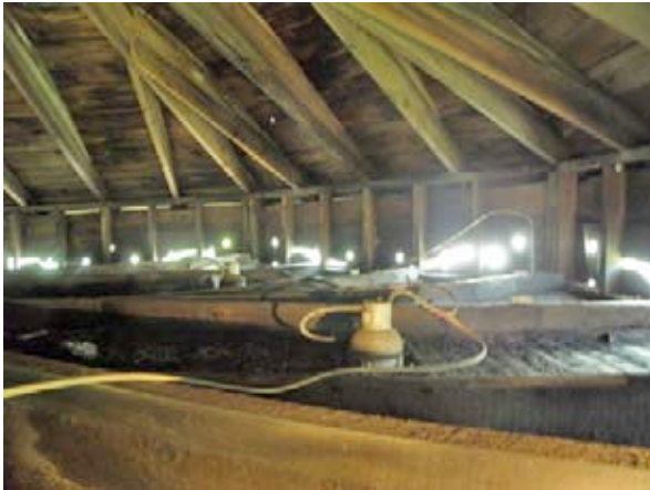
From the Ceiling Hatch Looking at the Southern Roof and Fascia
