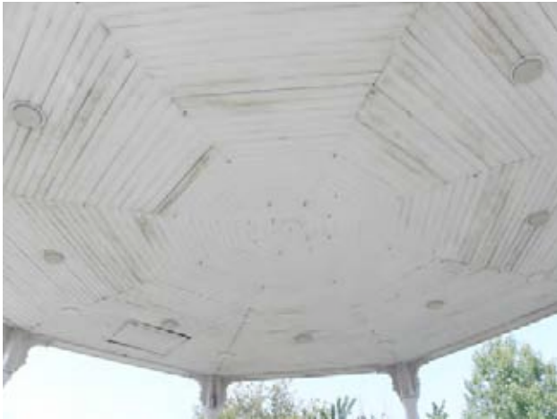
View of Ceiling Looking Northwest
