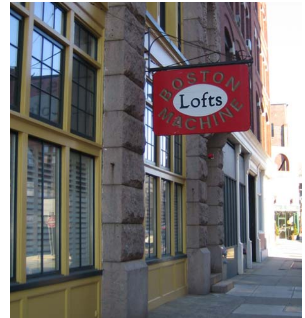
A RECENT DOWNTOWN LOFT CONVERSION
