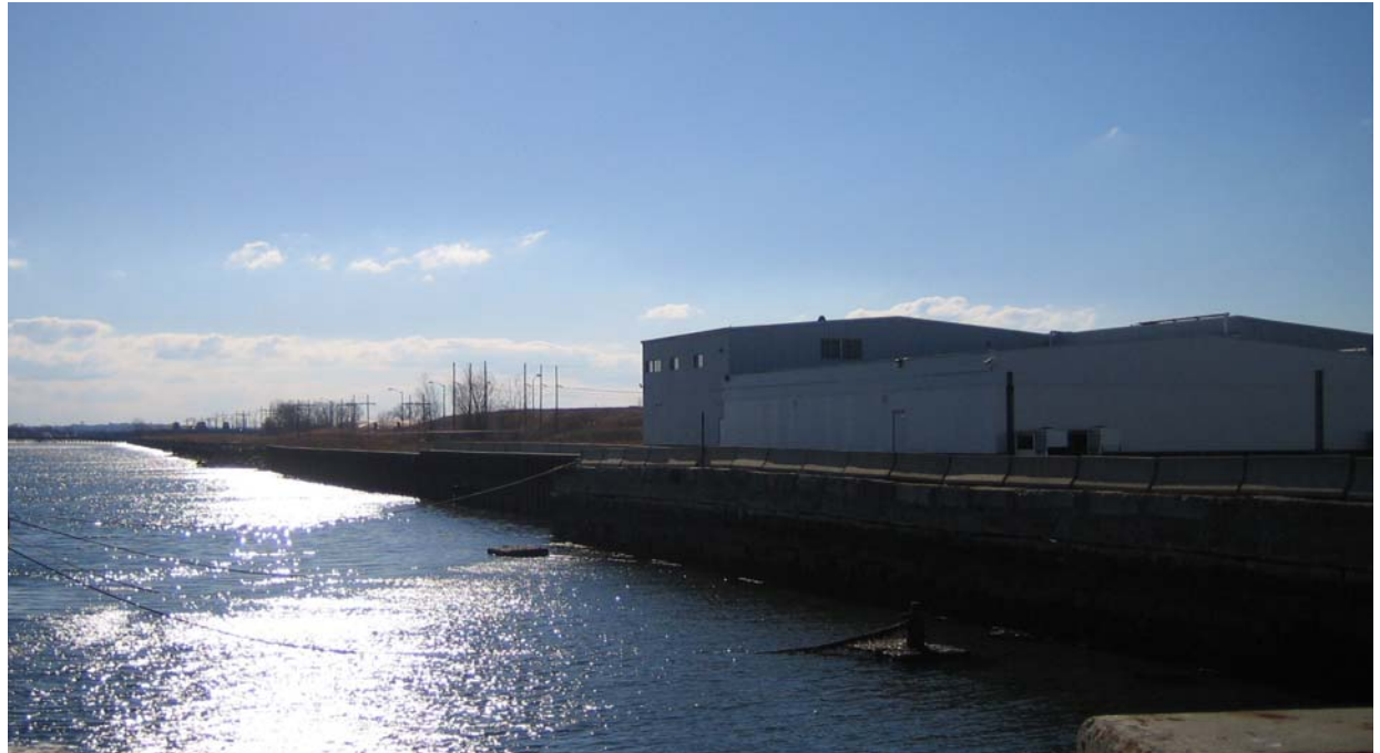
WATERFRONT SITE WHERE ADDITIONAL REMEDIATION WORK IS REQUIRED
